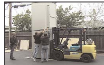
Above: The elevator being built outside Sunny's apartment building
